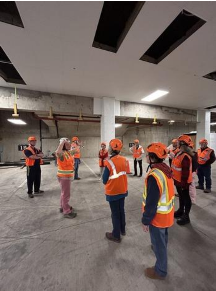
CAMS Manager, Jodie Jones, explains to volunteers how crews used fiber reinforced polymer (FRP) to strengthen columns in the Capitol garage.
